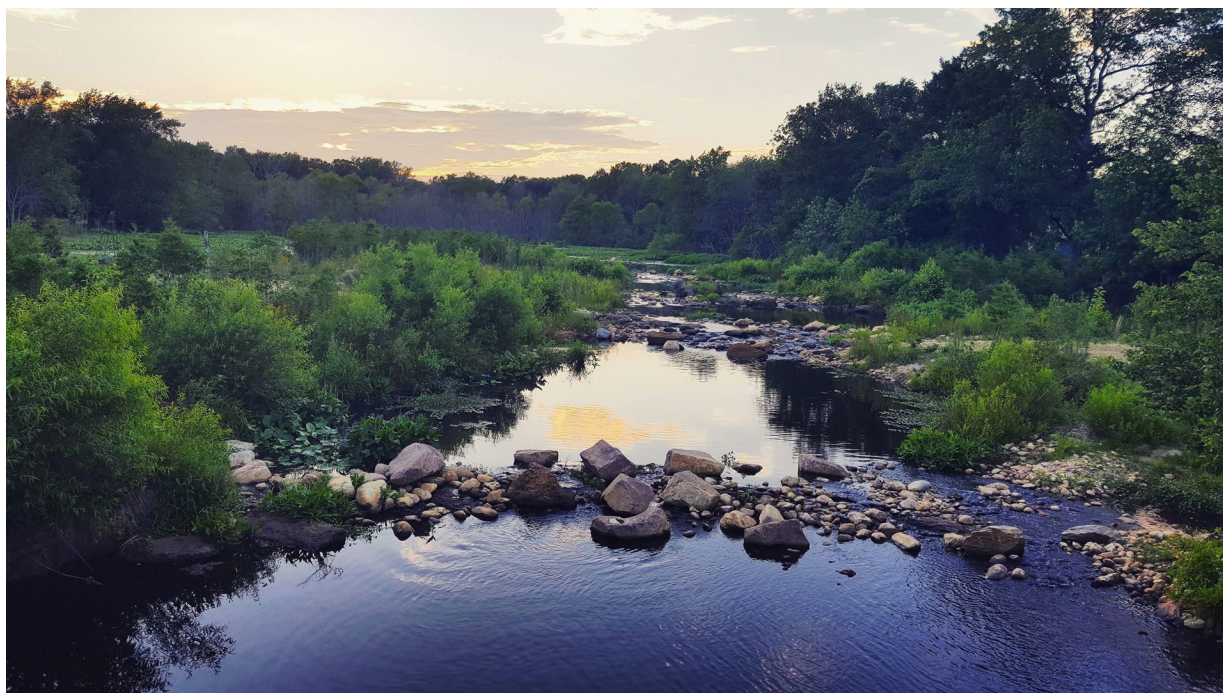
The removal of the Bishopville Dam provided opportunities for anadromous fish passage and provided a more ecologically robust and resilient stream and riparian corridor. Photo by Keith Pivonski.
