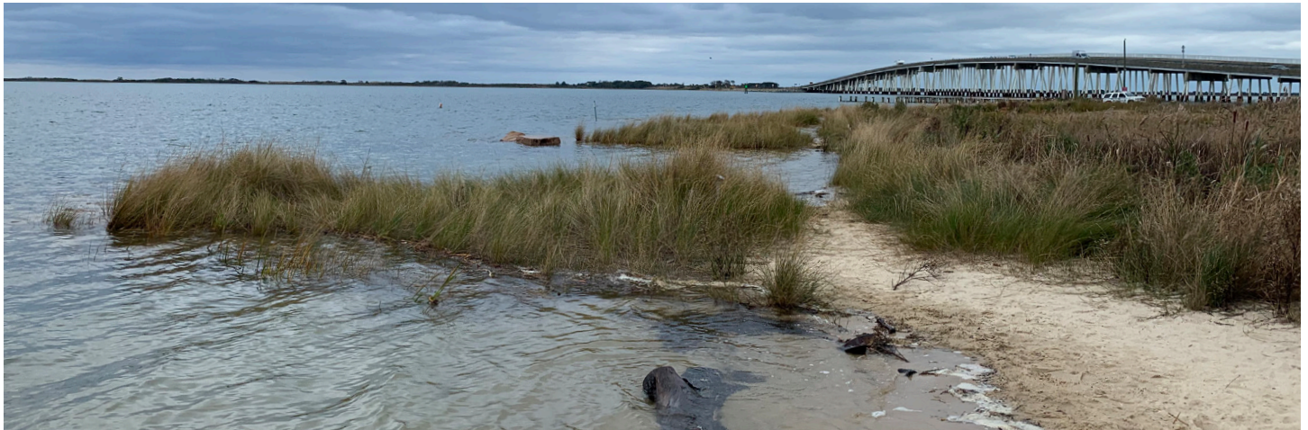
The Assateague Island State Park living shoreline 2 years after construction. Vegetated headlands diffuse and refract wave energy which maintain the quiescent coves. This shoreline project attracts nesting horseshoe crabs, diamondback terrapins, and marsh nesting birds such as willets. Photo by Roman Jesien.
