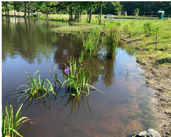
The Bainbridge Stormwater Retrofit shortly after completion. This project helps to address flooding and improve water quality in ocean Pines. Photo by Kevin Smith.
