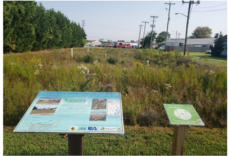
An old electrical transfer station was converted into a sand gravel wetland to collect and treat stormwater in a Berlin neighborhood prone to flooding. Photo by Roman Jesien.
