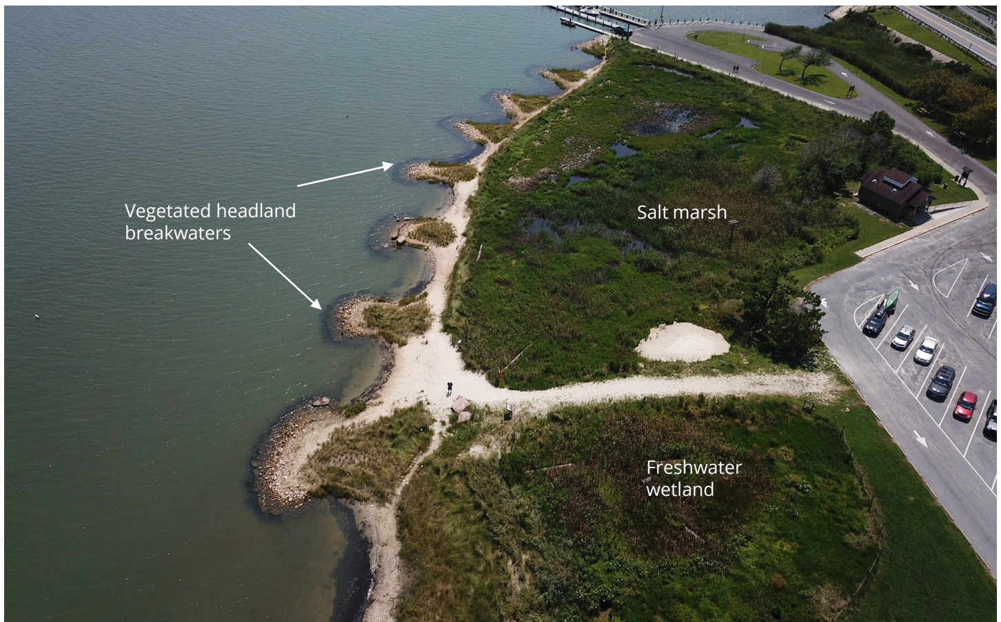
The living shoreline project near the Assateague State Park boat ramp. Eroding shoreline was enhanced with headlands and beaches that dissipate wave energy and a freshwater wetland that intercepts storm water. Photo by Roman Jesien.
