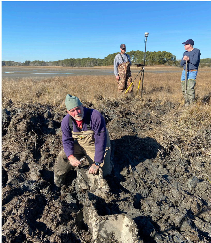
U.S. FWS, UMCES, and MCBP staff modify earthen and sheet pile plugs from mosquito ditches constructed in the early 1900's. Proper hydrology is critical to maintaining healthy and robust marsh ecosystems.
