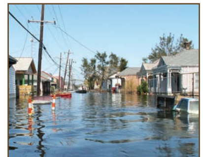
Flood damage following Hurricanes Katrina and Rita.
