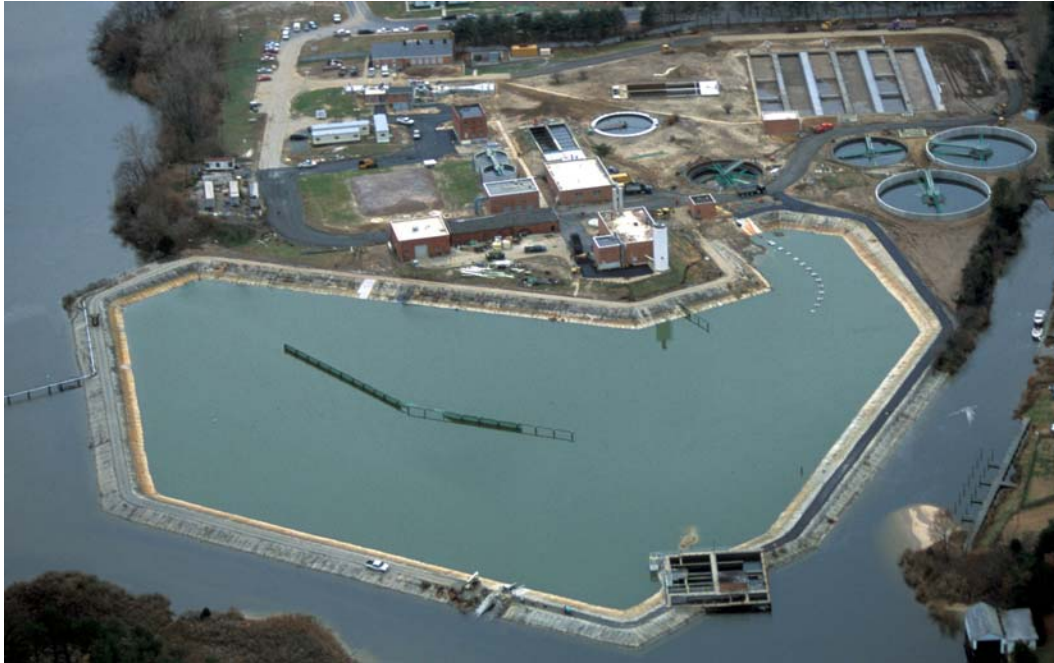
Plate 1. Cambridge Wastewater Treatment Plant. Sewage effluent has a high \delta^{15}\text{N} isotopic signature which can be detected by analyzing organisms inhabitant or incubated in the region.
