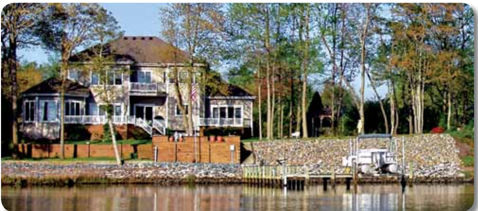
Hardened shorelines, such as this riprap along St. Martin River, offer fewer ecosystem benefits than natural shorelines.
