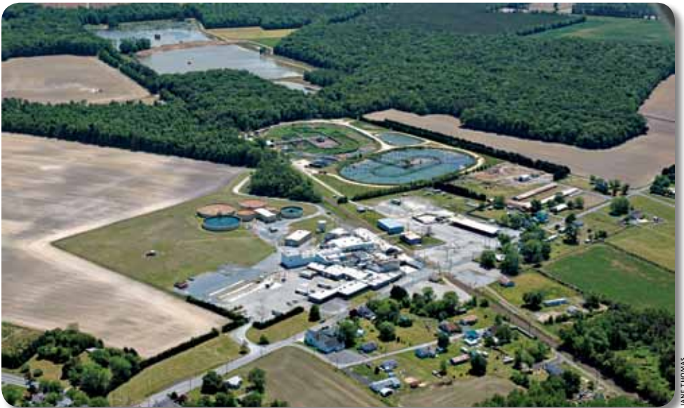
The former Perdue poultry processing plant on Middle Branch of Shingle Landing Prong, St. Martin River. This plant stopped production in September 2004; however, the wastewater treatment plant continued to operate for many months after that as the plant was cleaned and equipment removed.
