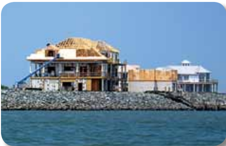
Riprap along the shoreline of a new development in Sinepuxent Bay.
