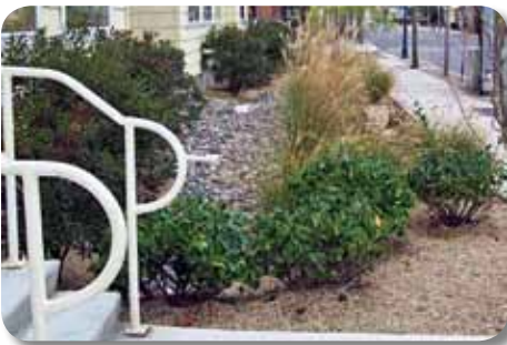
Bioretention in an urban environment. Bioretention utilizes soils and plants to remove pollutants from stormwater runoff.
