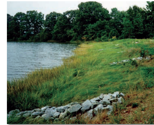
Sea-level rise contributes to the erosion of approximately 580 acres of shoreline per year. Maryland's Living Shoreline Protection Act of 2008 requires that living shoreline or non-structural shore protection practices be used wherever technologically and ecologically appropriate. Living shorelines provide erosion control benefits while also enhancing the natural shoreline habitat. They often allow for natural coastal processes to remain through the strategic placement of plants, stone, sand fill, and other structural and organic materials.
