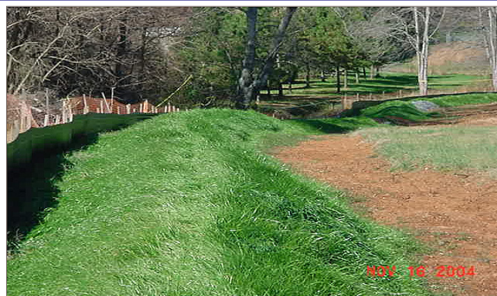
A grassy berm and silt fencing prevents stormwater runoff from this construction site.
