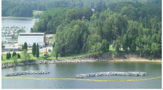
A stone revetment at the Naval Support Facility Patuxent River, Maryland replaced an existing deteriorating bulkhead. The yellow line floating in the water is a turbidity curtain that prevents sediments from moving downstream and decreasing water clarity.
