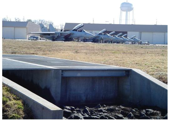
As the Department of Defense continues to support the Storm Water Directive, additional storm water management practices will be implemented on non-targeted public land parcels. This storm water runoff prevention system where wash rack water is captured in an oil/water separater is one method that could be used to reach the goals of the directive.
