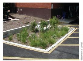
The Washington Navy Yard has installed many low impact development features, including this bioretention cell.
