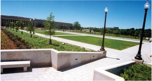
This parade ground is actually a green roof, which sits atop the Pentagon's Remote Delivery Facility. Green roofs are vegetated roofs that reduce impervious surfaces and decrease runoff.
