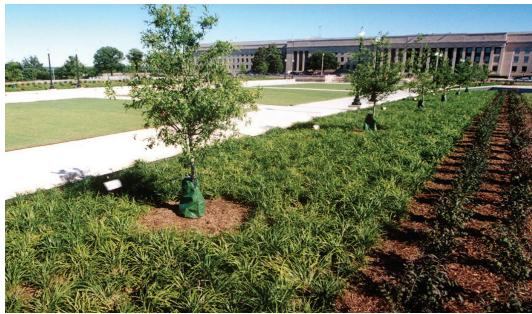
To construct this green roof at the Pentagon's Remote Delivery Facility, 12-18 inches of topsoil was placed on the roof to allow planting of grass and shrubs.
