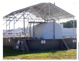
Secondary spill containment structures such as the concrete wall around this diesel tank at Naval Weapons Station Yorktown, Virginia are designed to capture any spills from the tank and allow for easy cleanup.
