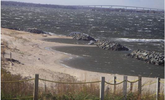
Stabilization of Fishing Point landfill using offshore breakwaters and beach grass plantings at Naval Support Facility Patuxent River, Maryland. Breakwaters and vegetation slow erosion and reduce sediment inputs to the Chesapeake Bay.
