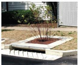
Washington Navy Yard Low Impact Development Demonstration Project on the Anacostia River. This project included the modification of the storm drain inlet.
