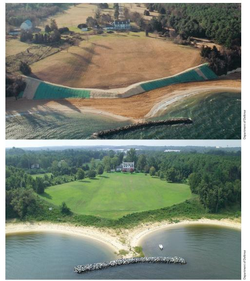
This project at Naval Support Facility Patuxent River, Maryland consisted of a system of four headland breakwaters with beach sands obtained from the adjacent sandy upland banks to create a series of stable pocket beaches. The project spans 2,200 feet of shoreline. *Top:* Quarters 'A' soon after construction. *Bottom:* Quarters 'A' one year later.
