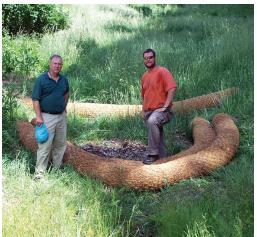
Jute logs are used to control erosion in a storm water swale at Navy Information Operations Command, Sugar Grove.
