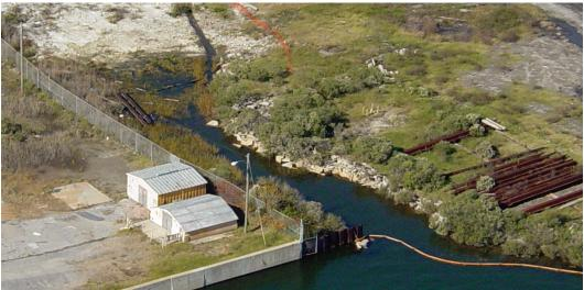
Prior to removal action, the settling lagoon at Norfolk Naval Shipyard, South Gate, contained calcium hydroxide sludge that was generated as a byproduct of acetylene gas production and heavy metals from paint chips in grit blast from small boat repair.
