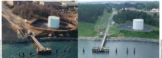
At the fuel pier at Naval Support Facility Patuxent River, Maryland, 410 linear feet of stone revetment were installed to protect the shoreline.
