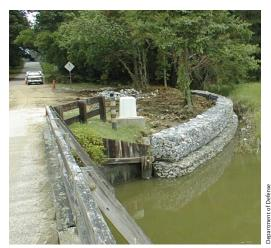
A shoreline stabilization structure at Felgates Crossing is made of gabion baskets, which are 'baskets' made of wire mesh and filled with piled stones.
