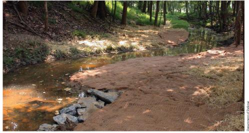
At the Naval Support Facility Indian Head, Maryland areas of erosion along this stream were reinforced with jute matting and grass seeding.
