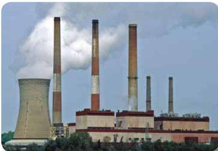
Power plants both nearby and far from Shenandoah produce air pollutants that impact park ecosystems.
