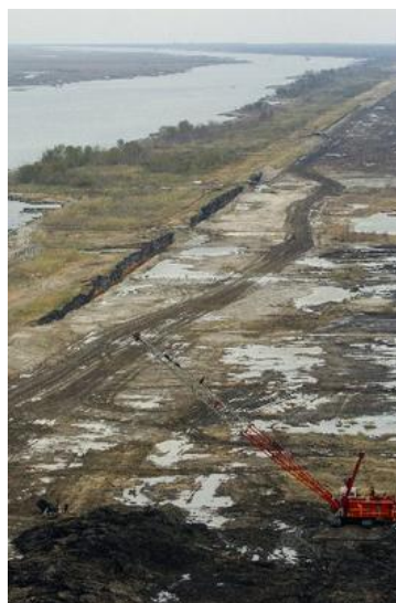
Rebuilding damaged levees along MRGO
