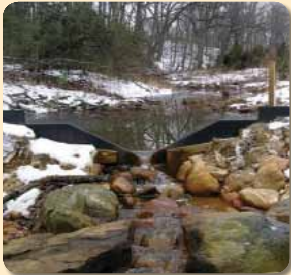
V-notch weir used to measure discharge at a stream restoration site.
