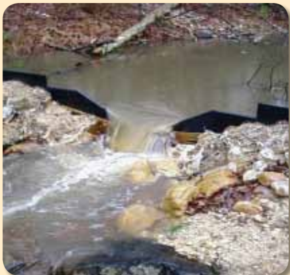
Stormflow event at the V-notch weir restoration site.
