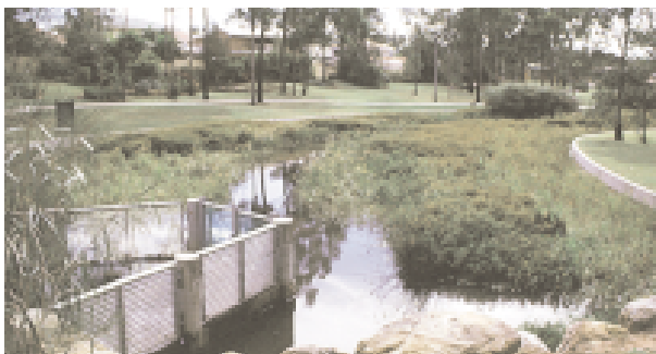
Stormwater quality improvement device (SQID)
