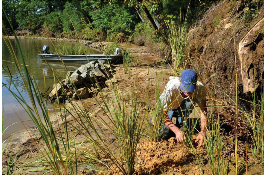
Living shoreline project on Church Creek will help to stabilize the shoreline and allow swamp, shoreline, and floodplain forest species to migrate to higher elevations.
