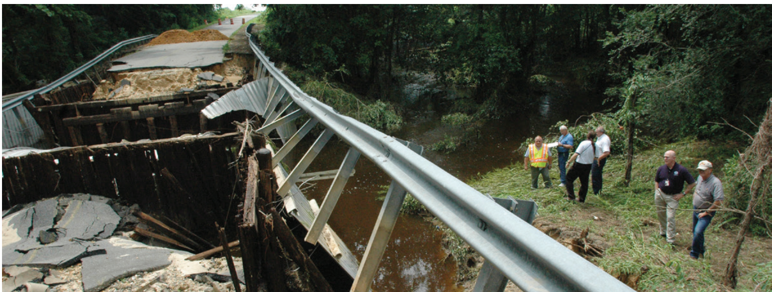
Dorchester County, Md., June 2, 2006—Members of a Preliminary Damage Assessment Team (PDA) survey the damage to this road and bridge on Maryland’s eastern shore. The teams, made up of State, County, and FEMA, evaluate damage and make a recommendation for a Federal disaster declaration. The damage to Maryland’s roads, bridges, and housing was caused by severe rain and flooding.
