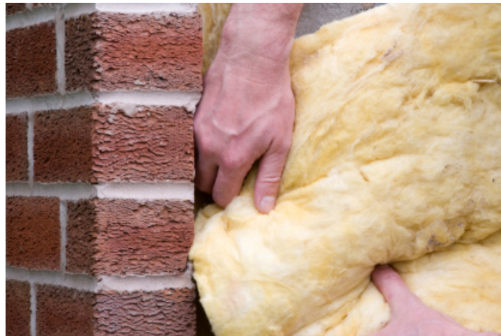
A worker installing insulation to improve energy efficiency.
