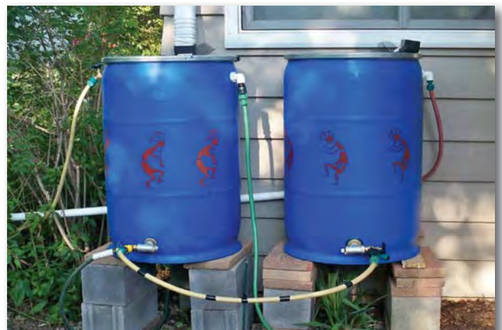
Rain barrels help hold back stormwater and reduce combined sewer discharges in our urban areas.
