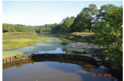
A notch cut in the dam (seen far right) allowed the water to slowly decant while retaining sediments in the pond. This project is now close to completion.
