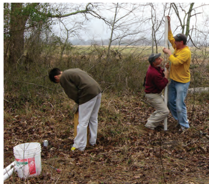
The installation of wells to allow monitoring of groundwater gives information about the concentration of nutrients in the groundwater. Photo by Roman Jesien.
