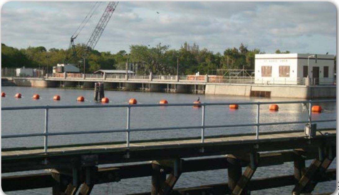
The flow of water across the south Florida landscape has been modified into a series of canals with structures that control the amount of water delivered to estuaries and coastal areas (St. Lucie Lock in the Okeechobee waterway, Martin County).
