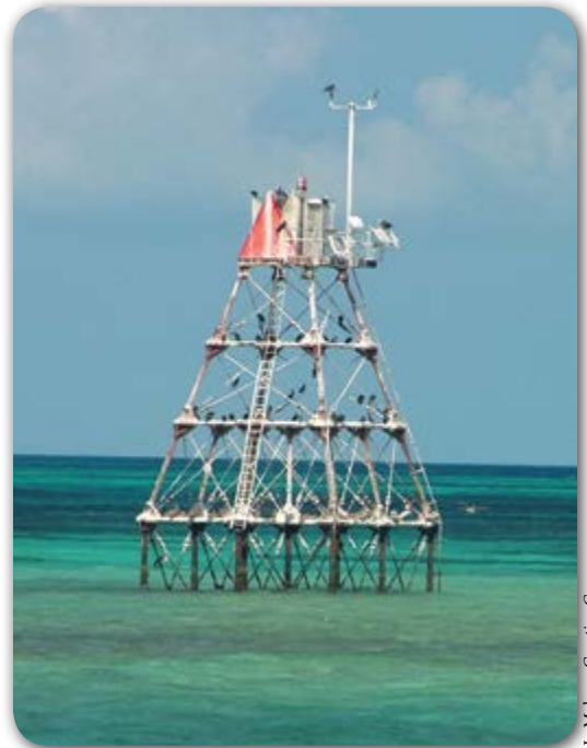
Real-time oceanographic data are collected from instruments fastened to the Molasses Reef Lighthouse and transmitted by satellite to the NOAA Atlantic Oceanographic and Meteorological Laboratory for analysis.
