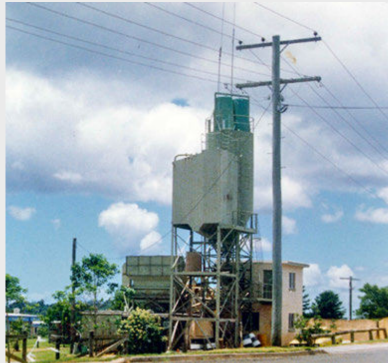
The Sellars Holding Concrete Batching Plant situated next to Maleny State High School in 1990.
