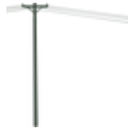
Energy: power line
