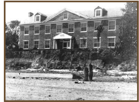
Erosion damage at the UMCES Chesapeake Biological Laboratory in Solomons after the 1933 hurricane. Image courtesy Calvert Marine Museum Archives.
