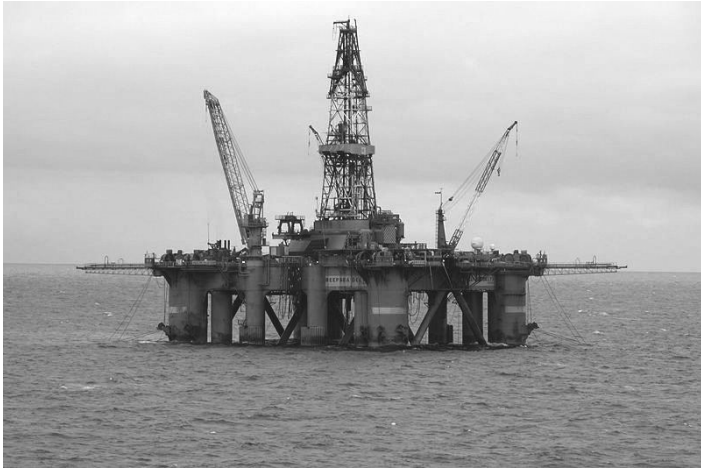
Fig. 5. Oil drilling platform Harvest operating 11 km (~7 mi) off the coast of California in 200 m (650 ft) of water. Source: Minerals Management Service, U.S. Interior Department. (As noted in footnote 3 of Chapter II, drilling had been banned for sometime from all sites such as this though they could pump from oil straits that had already been reached.)
