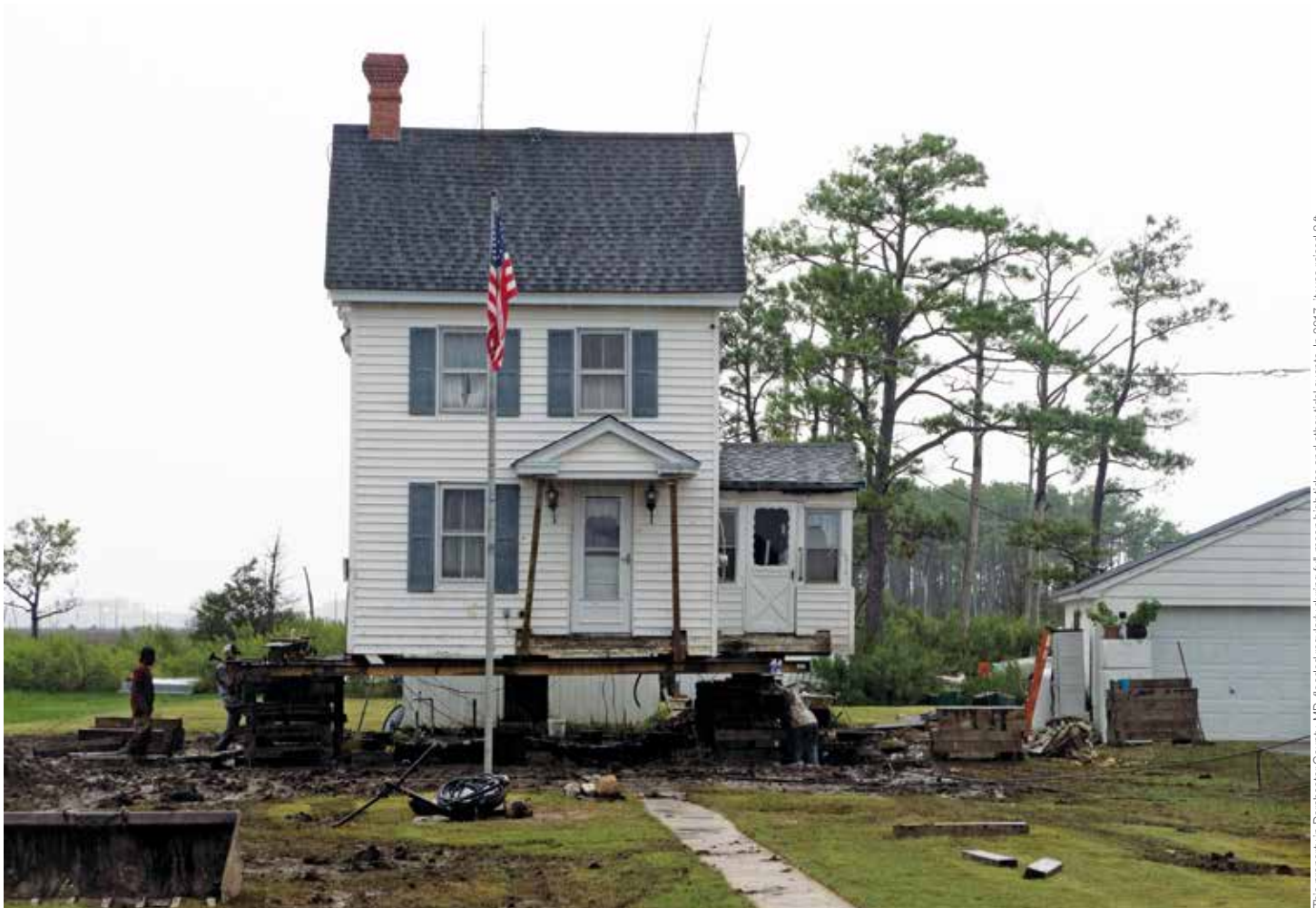
This property in Dorchester County, MD, flooded regularly during full-moon high tides and other tidal events. In 2017, it was raised 8 ft. David Harp/ChesapeakePhotos.Corn.
