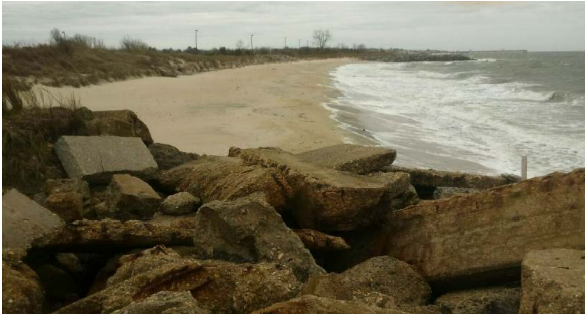
Groins along the beach on the Chesapeake Bay, Virginia (Photo credit: Maggie Latimer, University of Richmond).
