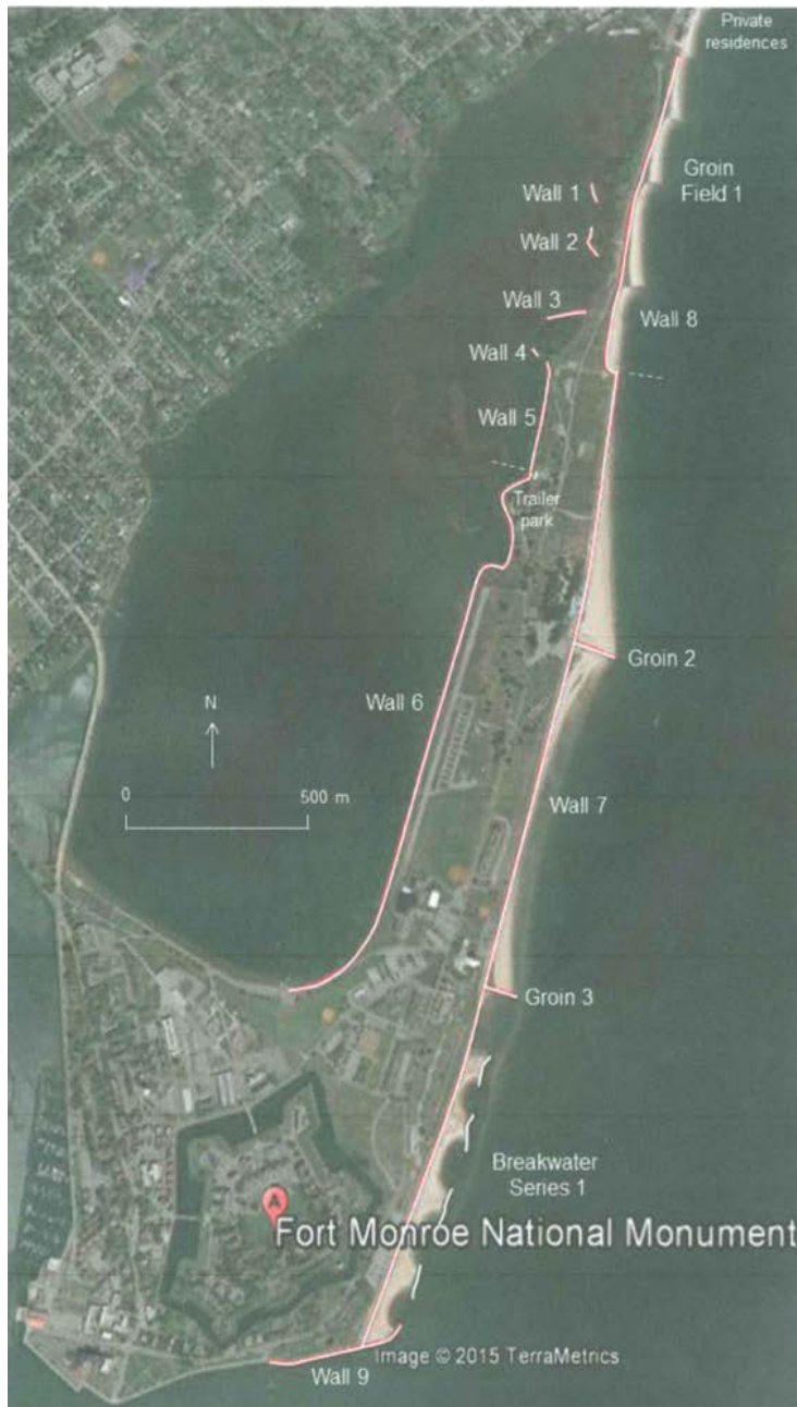
Figure 4-26. Walls and groins along Fort Monroe National Monument's shoreline (Figure from Nordstrom and Jackson 2015).
