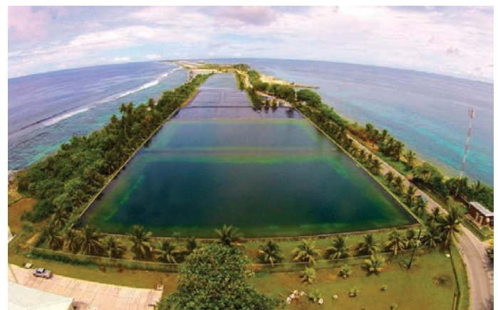
The freshwater storage reservoir on Majuro Atoll. Photo from Majuro Water and Sewer Company via FEMA.
