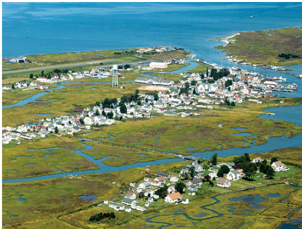
Virginia's Eastern Shore is vulnerable to flooding.
