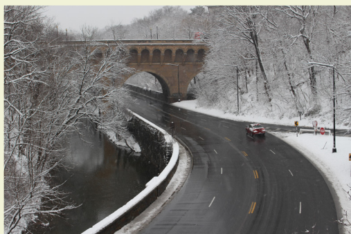
The Q Street bridge in winter.
