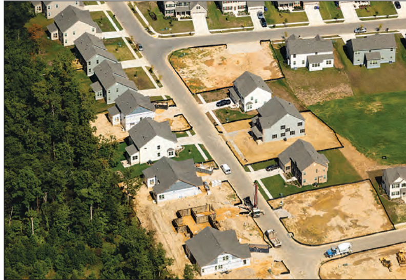
A partly completed residential development borders forested land in Waldorf, Maryland. Courtesy of the Chesapeake Bay Program, used with permission.
