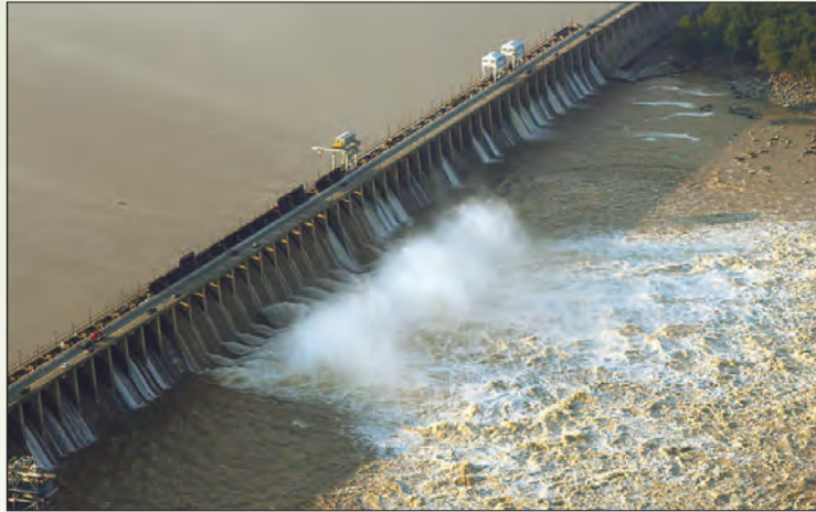
Figure 4.S1. View of the Conowingo Dam on the Susquehanna River in the aftermath of tropical storm Lee. Photograph taken at 4:30 p.m. on September 12, 2011. Streamflow at the time was 220,000 cubic feet per second. Peak streamflow for the flood was 778,000 cubic feet per second at 4:00 a.m. on September 9, 2011. Photograph by Wendy McPherson, U.S. Geological Survey.
