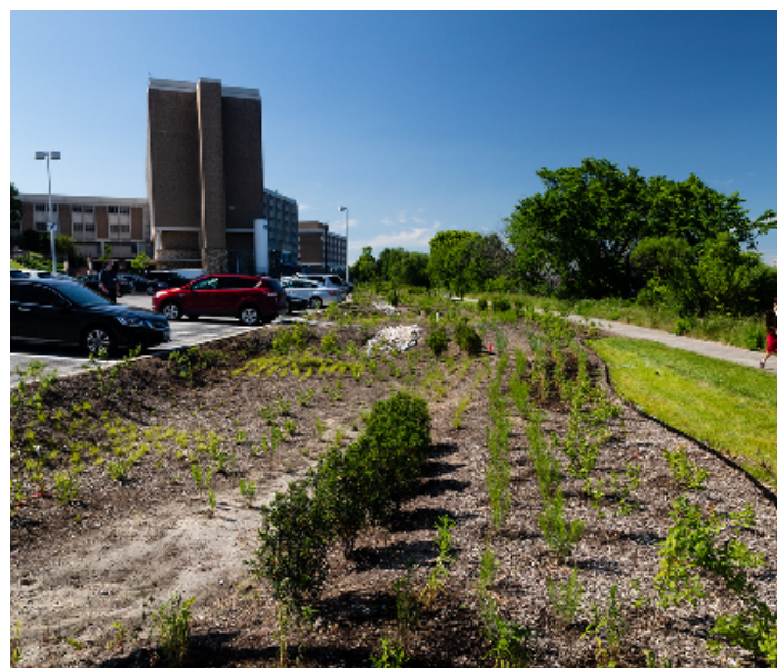
A natural buffer is planted on the side of MedStar Hospital in South Baltimore. This is a successful example of a collaborative green infrastructure project.
