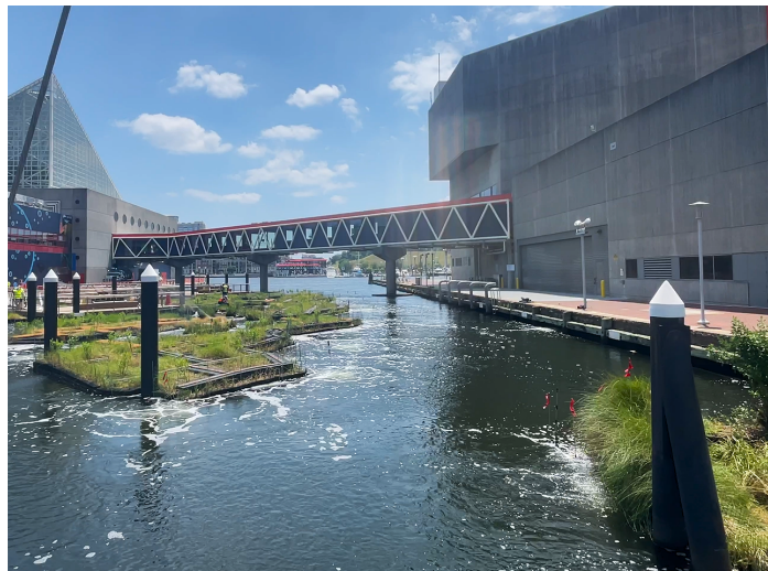
Floating wetlands installation at the National Aquarium in Baltimore Harbor as of summer 2024. These planted areas improve habitat, water quality, and the general environment. Otters have been documented using this new greenspace.
