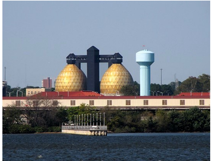
Back River Waste Water Treatment Plant is located in Baltimore. They are also known as the "golden eggs".
