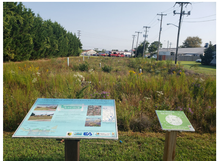
An old electrical transfer station was converted into a submerged gravel wetland to collect and treat stormwater in a Berlin neighborhood prone to flooding. Photo by MCBP staff.
