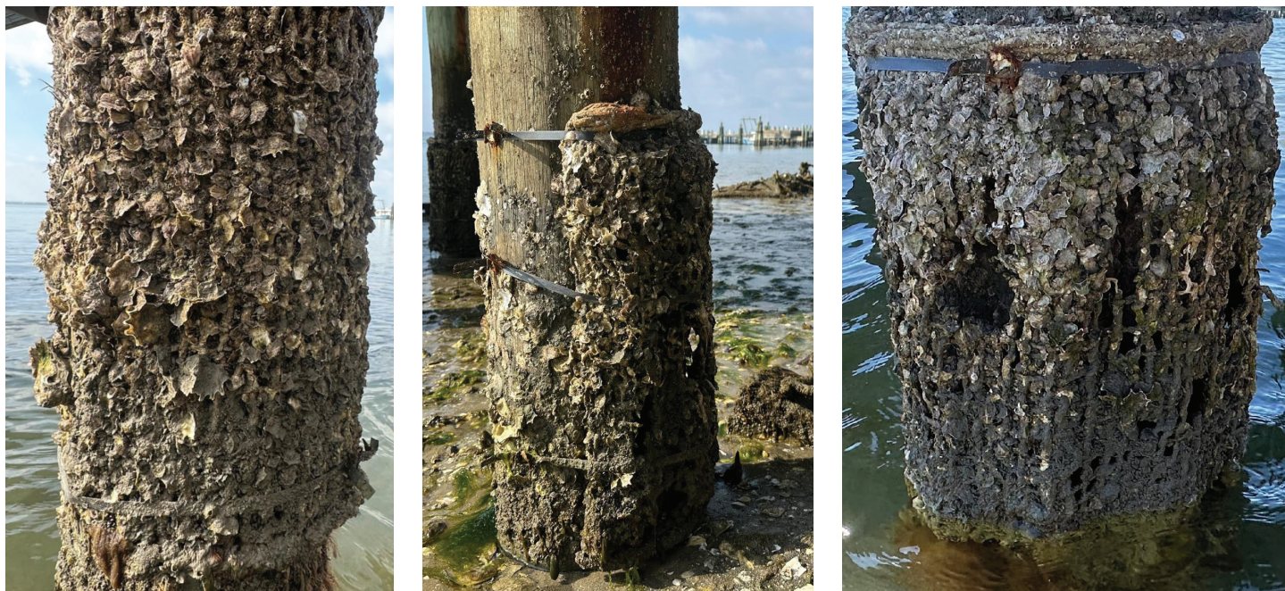
Figure 4A.2 Oyster Catcher™ piling cuff installed in Bogue Sound, Morehead City, NC in February 2024, and photographed a year later. Photos courtesy of Niels Lindquist.
