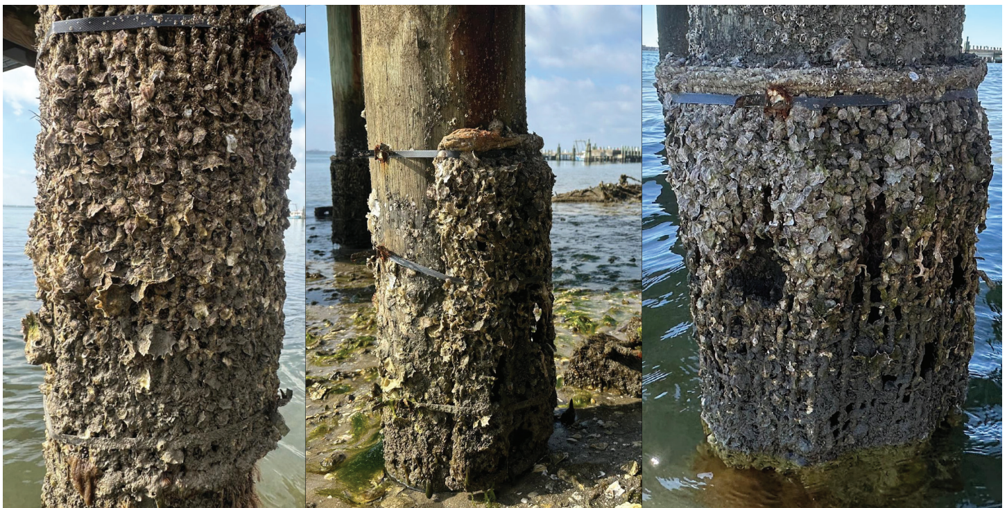
Oyster Catcher™ piling cuff installed in Bogue Sound, Morehead City, NC in February 2024, and photographed a year later. Photo courtesy of Niels Lindquist.
